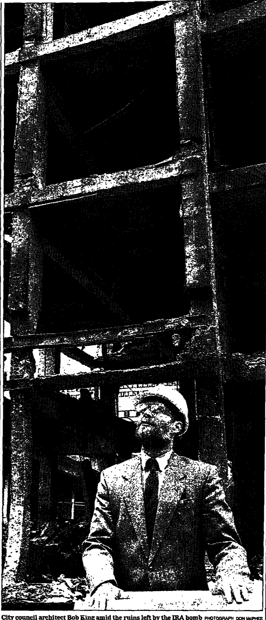
City Council architect Bob King amid the ruins left by the IRA bomb. PHOTOGRAPH DON MCPHEE
